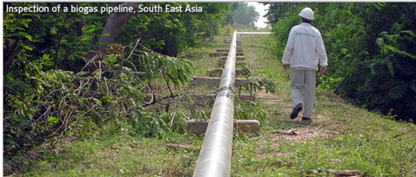
Inspection of a biogas pipeline, South East Asia
